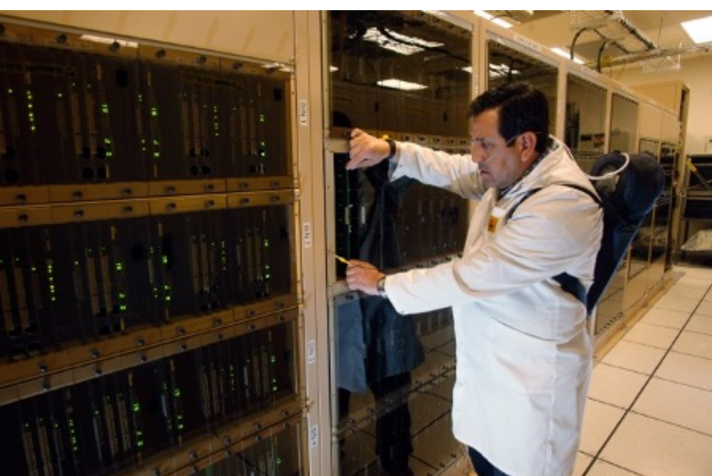
While the 1st generation correlator is hosted in the Array Operations Building at 5000 m of altitude, a new correlator facility to host ALMA-TALON will be set up at 3000m at the Operations Support facility. Carlos Padilla, NRAO/AUI/NSF
